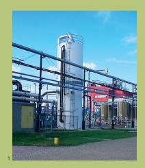
After four years of successes and setbacks for Rozenburg's Environmental Project, a new biological off-gas purification unit has been installed at the Lucite<sup>®</sup> Diakon<sup>®</sup> plant and early signs look extremely positive. Called a Moving Bed Trickling Filter (MBTF) unit, this new piece of equipment replaces the Bio Trickling Filter (BTU) unit, which we reported about in GF, June 2004.
